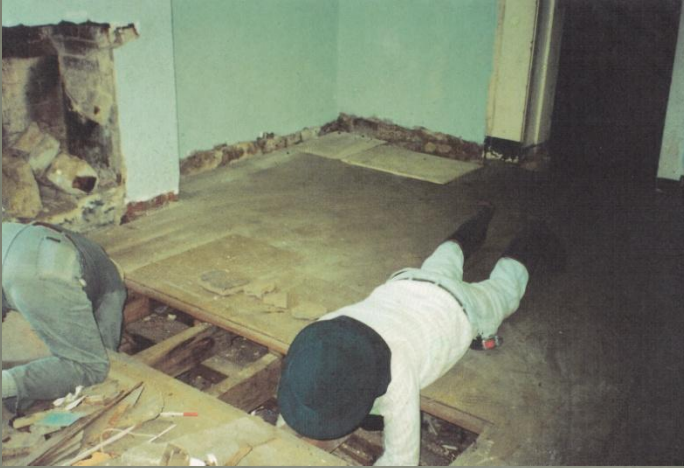
Repairing under floor problems
